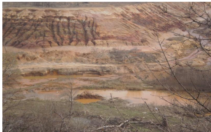
Figure 18: Industrial waste landfill with erosion faults on the river Ibar bank in Kosovo*
