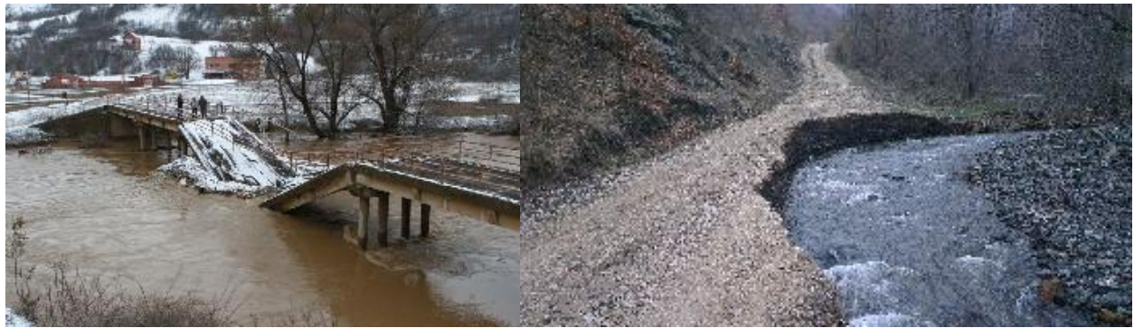
Figure 17: Floods in Kosovo* in the year 2013; Broken bridge in Kutnje (left); Damaged road (right)
