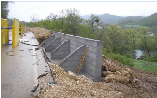
Figure 52: Construction of retaining wall.
