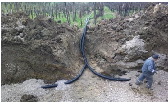
Figure 53: Drainage of landslides as permanent measures of protection.
